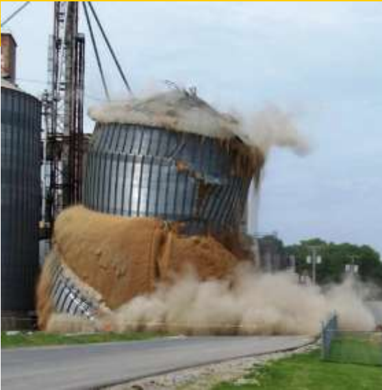
Bridging transfers load to the bin wall
